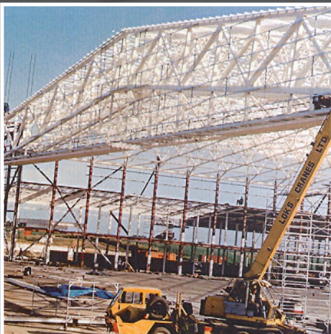
Space Frame Roof and building assembly - 1100mt - Air Pacific, Fiji
